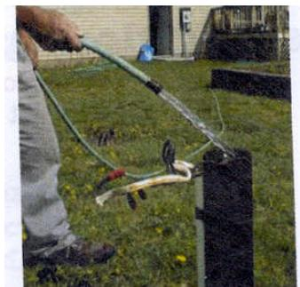
After the water has run clear for a while turn on **all** faucets connected to the well throughout the house and outside the house, including the hot water faucets. Make sure to turn on faucets that rarely or never get used, especially yard hydrants and outside spigots. Remember to run water into the washing machine and flush all toilets. Run the water until the chlorine smell is detected.
